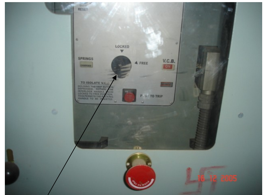
Lock/Free s/w for VC in/out should trip VC mechanically ( Standard safety Features)
