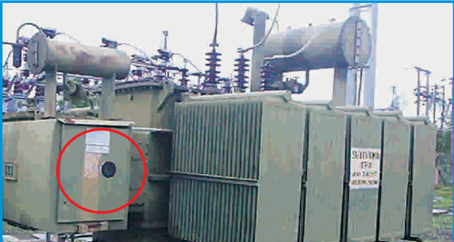
Transformer On line tap changer( OLTC)
