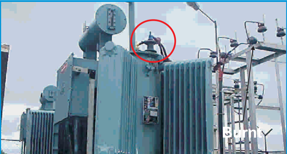
Transformer Manual tap changer
